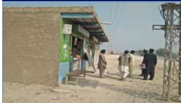
Plate 32: A view of affected structure and Electric poles at Starting point of Kandhkot – Kashmir Section near Jamia Masjid Khawaja Ghreeb Nawaz.
