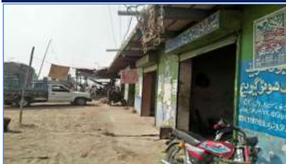
Plate 31: A view of affected structure at Starting point of Kandhkot – Kashmir Section near Jamia Masjid Khawaja Ghreeb Nawaz.
