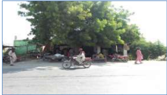
Plate 12: A view of affected Structure at Jahan Khan Bangwar, Kashmore
