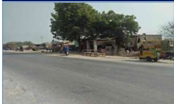
Plate 30: A view of affected structure at Goth Jahan Khan Bangwar.
