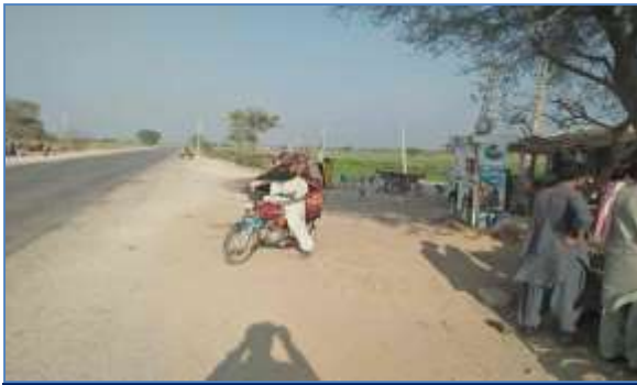
Plate 43: A view of affected temporary structures at Mando Khan Jakhriani, Kashmir.
