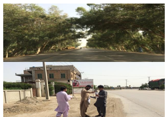
Plate 30: Photographs showing the end point of the road alignment at Rajanpur. In addition, above photograph showing the impact on the trees along the existing road, which requires to be cut-down.
