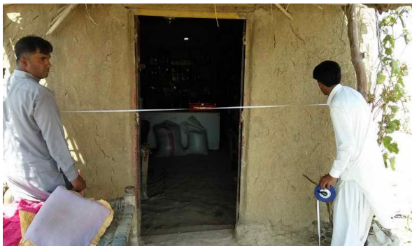
Plate 41: A view of affected structure located within the road RoW Kashmore – Rojhan Section.
