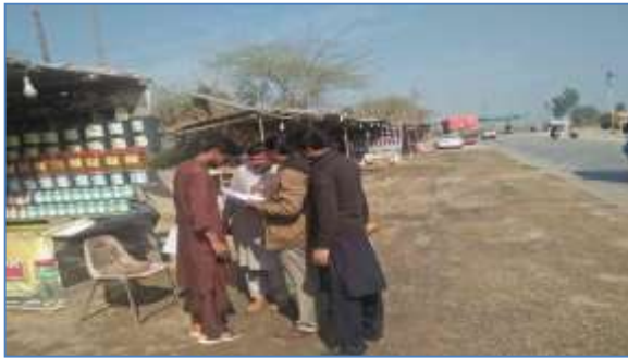
Plate 33: A view of Joint validation of affected thatched shed at 45+000 Shikarpur.
