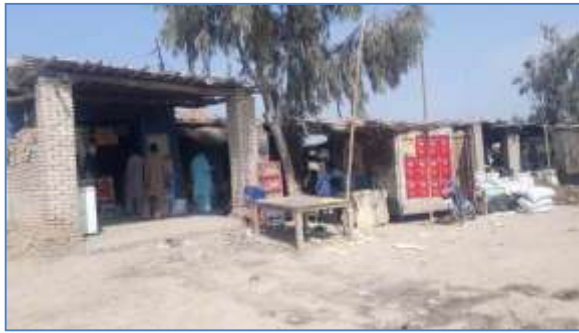
Plate 17: A view of affected Structures at Shikarpur .
