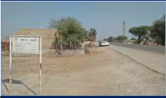
Plate 46: A view of affected structure at Machi Bindo, UC Jamal, Shikarpur
