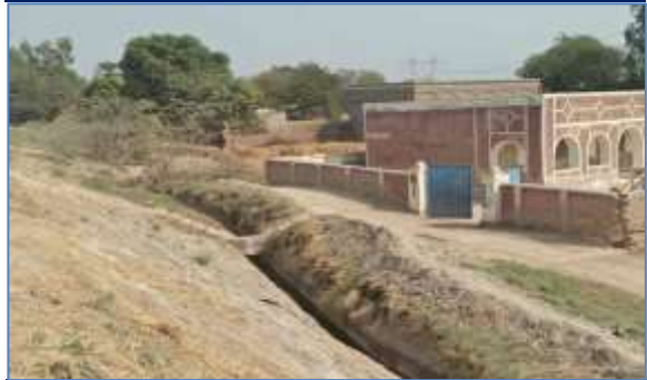
Plate 52: A view of right side affected School at Chainage 98+400, Tangwani Stop.
