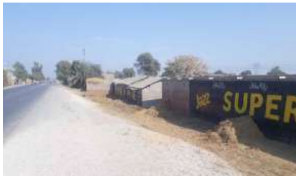
Plate 19: A view of affected Structures at Machi Bunda, Shikarpur – Kandhkot Section
