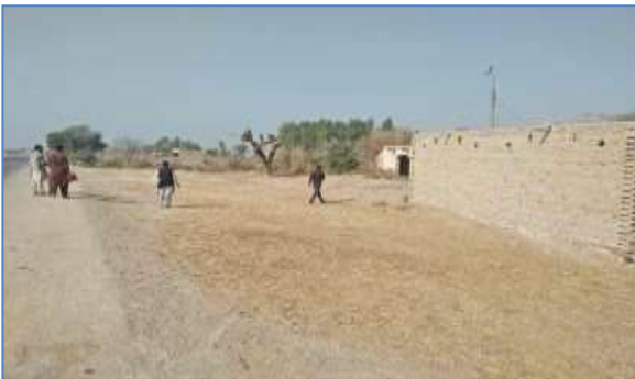
Plate 35: A view of affected structure left side at Goth Qadir Bux, Shikarpur
