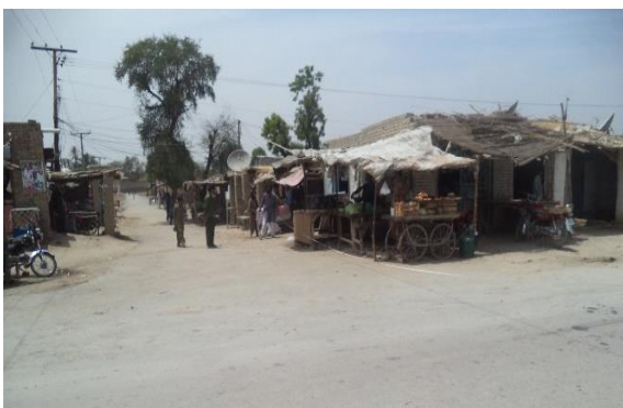
Plate 52: View of commercial structures located within the limit of ROW, which need to be shifted.
