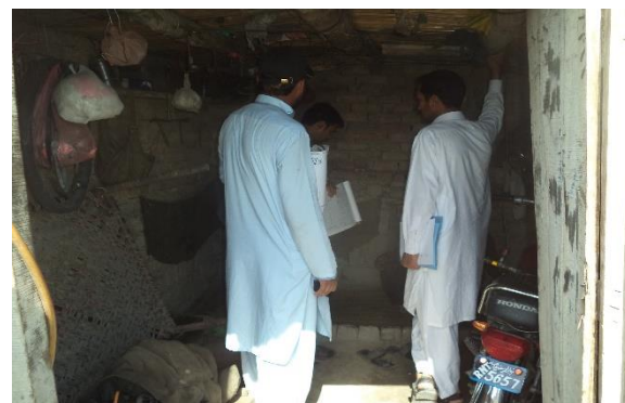
Plate 53 A view of inside of the affected business structure found within the RoW along the road alignment.
