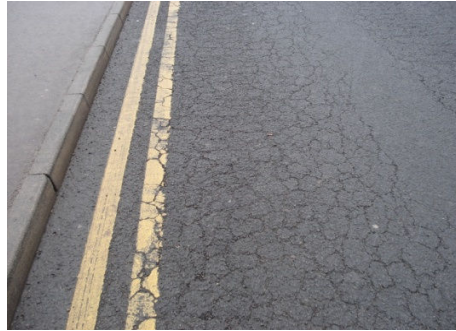
Fatigue Cracking
