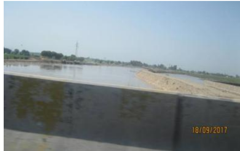
Canal bridge at Karam Pur Area
