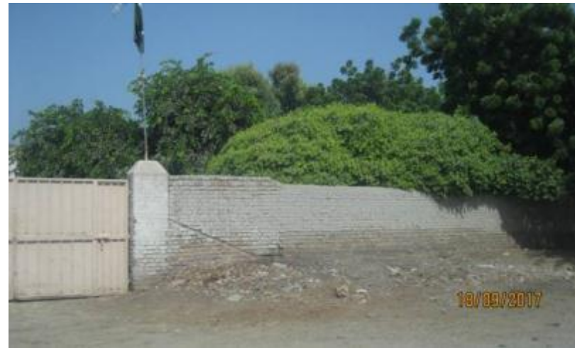
Rice mill area across the N-55 highway at Khan Pur Area
