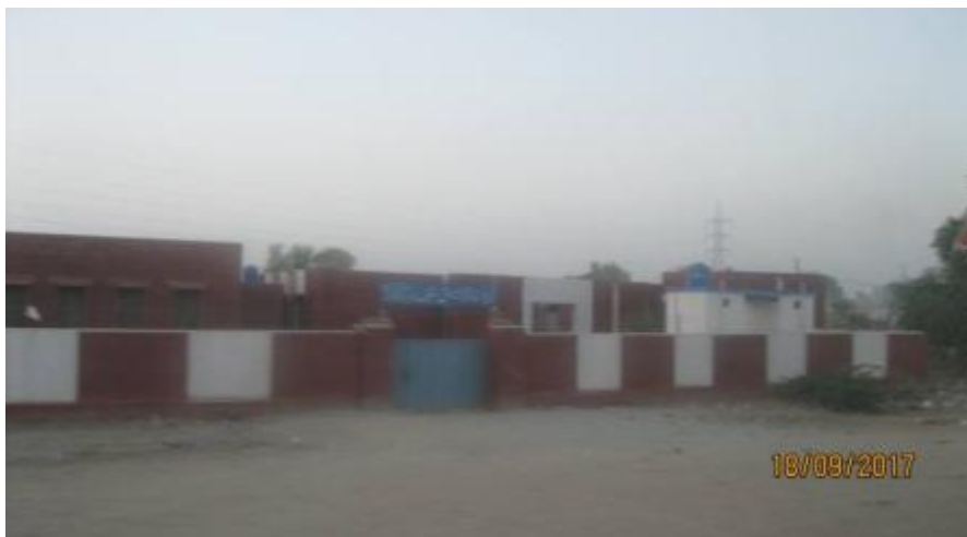
School Located adjacent to ROW (at Miran Pur City Area )
