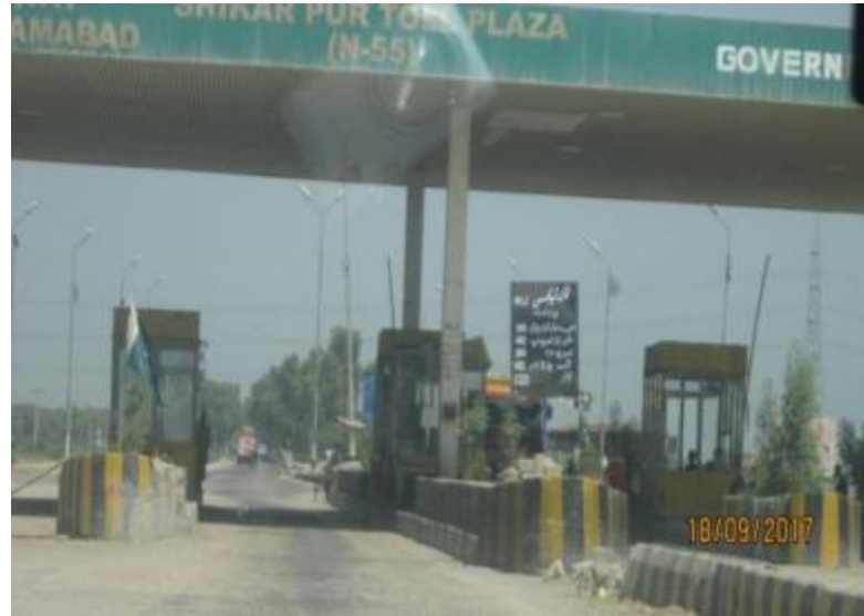
Toll Plaza, Shikar Pur
