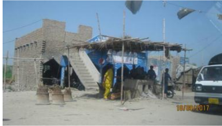
Commercial structures along the N-55 at Faizo Laro (Ghot Dado Khan)
