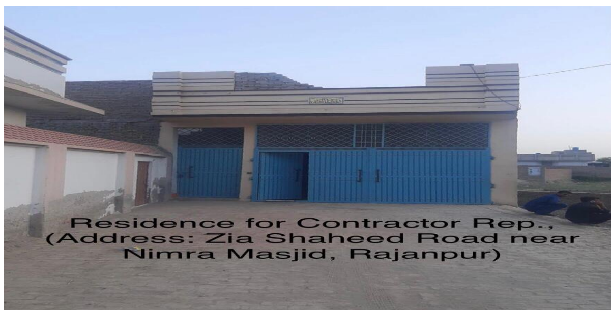
Figure 3-2: Kanal furnished building for accommodation for site staff in Rajanpur
