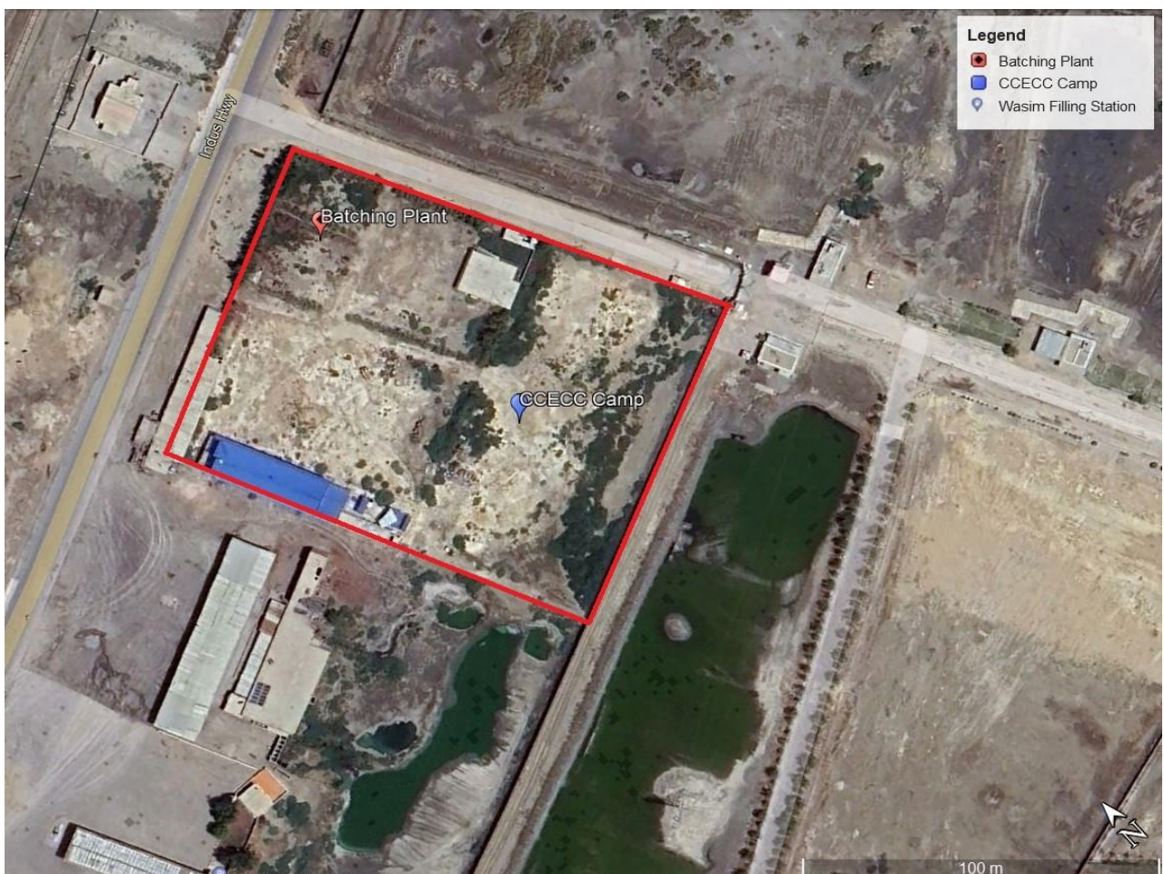
Figure 3-2 : Camp and Batching plant site before construction
